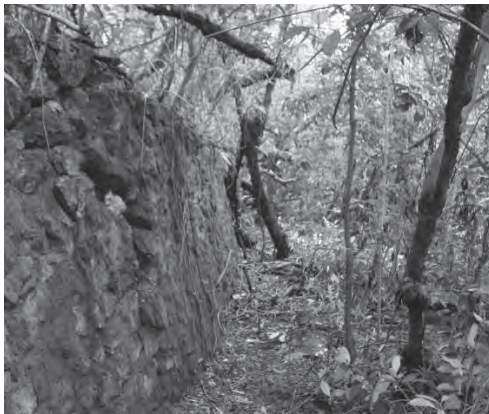
Rock wall, resource #2 on aerial overlay.
