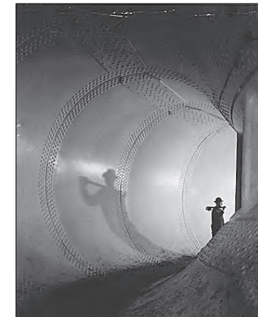
A Tennessee Valley Authority hydroelectric dam under construction. Courtesy of Franklin D. Roosevelt Library.
