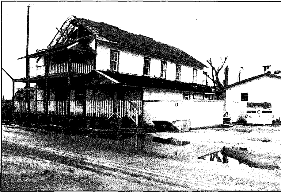
(Top) William Anderson General Merchandise Store (1912), Goulds. This frame vernacular building was recently rehabilitated as a restaurant. It sustained severe structural damage.
