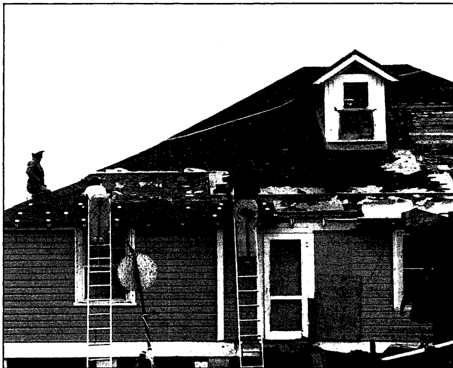
The Florida Pioneer Museum, originally a 1904 Florida East Coast Railway station agent's house, is shown here as Historical Museum staff members begin repairs and cleanup.
