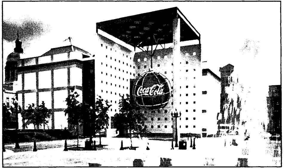
The World of Coca-Cola, adjacent to Underground Atlanta.
