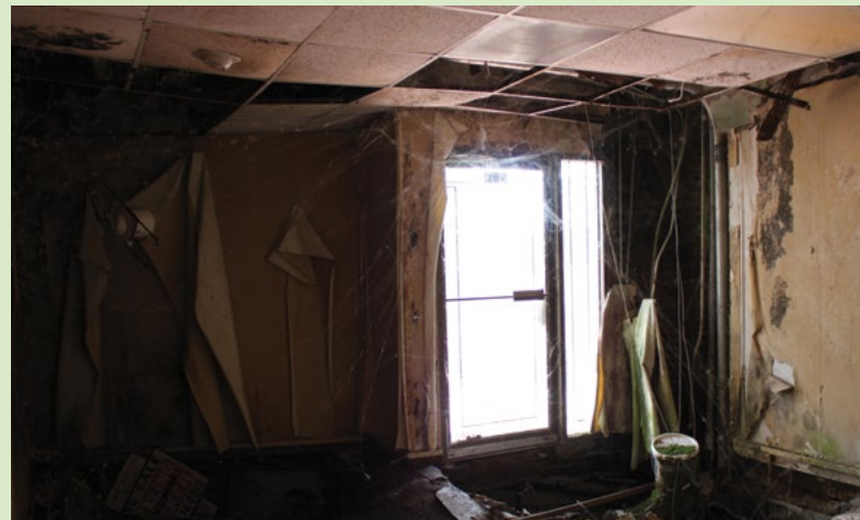
Interior, Capricorn Office Building. The water damage throughout the building was so severe that there were several collapsed sections of floor and some missing roof. In 2015, a local developer interested in saving this building and its history purchased the structure and planned to rehabilitate it using historic tax credits. Because of the façade, the building is currently non-contributing. Due to the structure’s deteriorated state, Georgia’s Historic Preservation Division determined it did not have enough material integrity to qualify for National Register listing. Georgia’s Historic Preservation Division did suggest that the building could qualify for the Georgia Register of Historic Places with an integrity of feel if it was restored to a “1970s” interior appearance. Image courtesy of Historic Macon Foundation.
