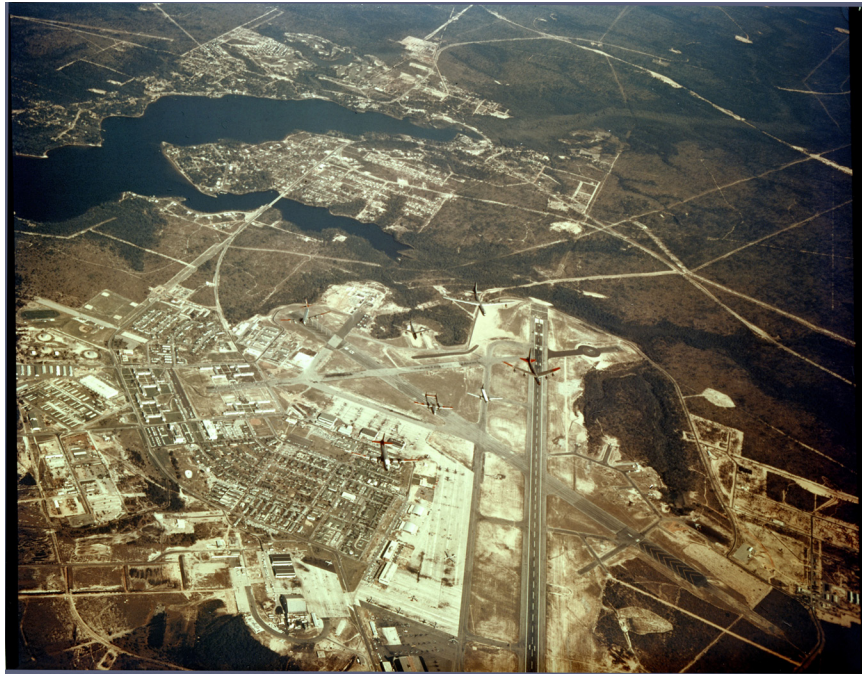
Figure 1.1: Aerial View of Eglin Air Force Base, Florida. Courtesy National Archives, NAID: 176246632
