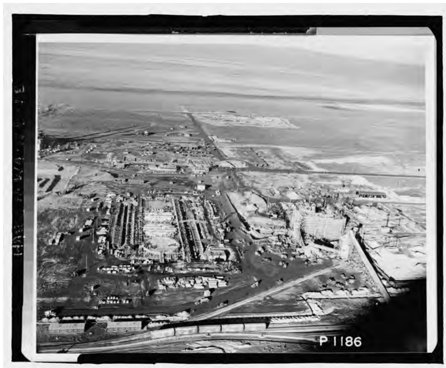
Figure 1.3: Aerial view of the 100-B Area of the Hanford Site under construction in January 1944, Richland, Washington. Courtesy Library of Congress
