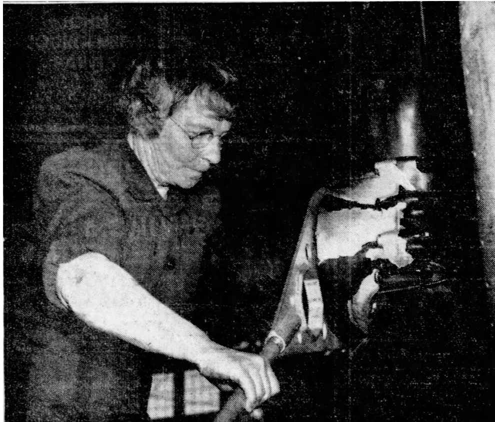
Figure 28: Neal Forsling, shown removing the dome of a Hamilton hydromatic propeller at the 348th Sub-Depot, Casper Air Base. U.S. Army Air Forces from The Casper Star-Tribune , Sept. 30, 1943. (Also archived in Elizabeth "Neal" Forsling Newspapers and Jean Gallatin Ogilbee Photo Album, NCA 01.v.2024.08 WyCaC US. Casper College Archives and Special Collections)
