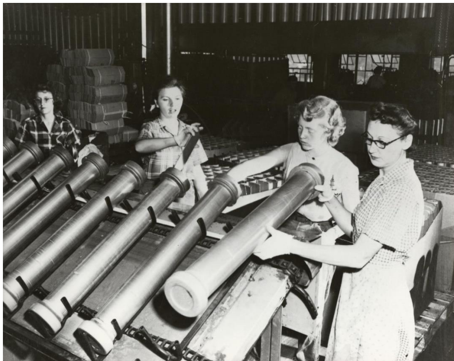
Figure 12: Women working on aluminum three-inch shell canisters on an Aluminum Goods Manufacturing Company assembly line. These canisters were used to transport artillery shells. (Credit: P82-64-12, Wisconsin Maritime Museum Collection, copy and reuse restrictions apply.)
