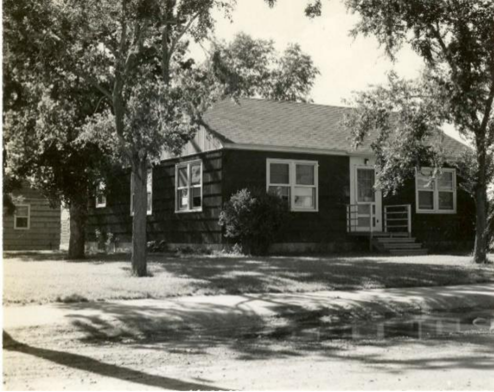
Figure 5: The house captured above is one of the famous alphabet houses (model H, photograph likely taken in mid 1950s) and designed for permanent professional, primarily white, workers. (Credit: Courtesy of the Hanford History Project)
