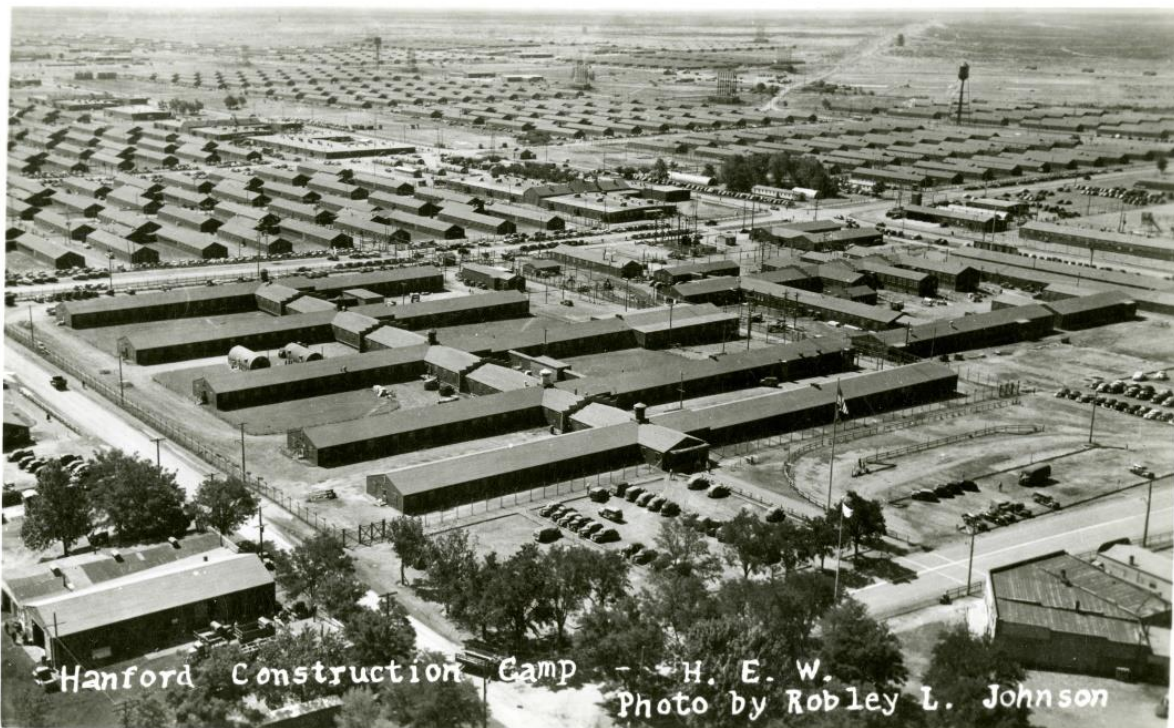
Figure 4: Hanford Construction Camp, circa 1944. When plutonium production began, the camp was dismantled. (Credit: Courtesy of the Hanford History Project)
