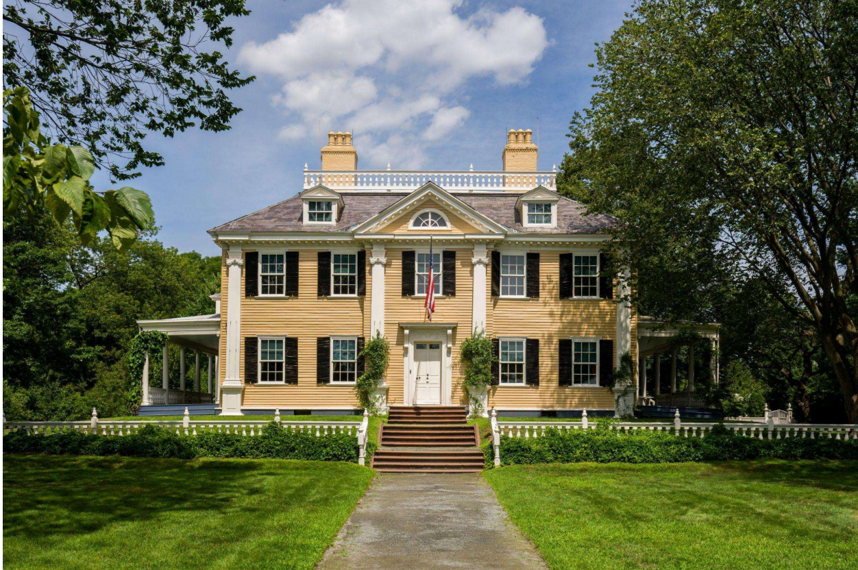
Figure 2. Front facade of the Longfellow House—Washington’s Headquarters National Historic Site in late summer, the structure’s symmetry characteristic of the Georgian style of architecture. Reproduced by permission of the National Park Service and the artist, Photography Rhode Island, James. P. Jones.
