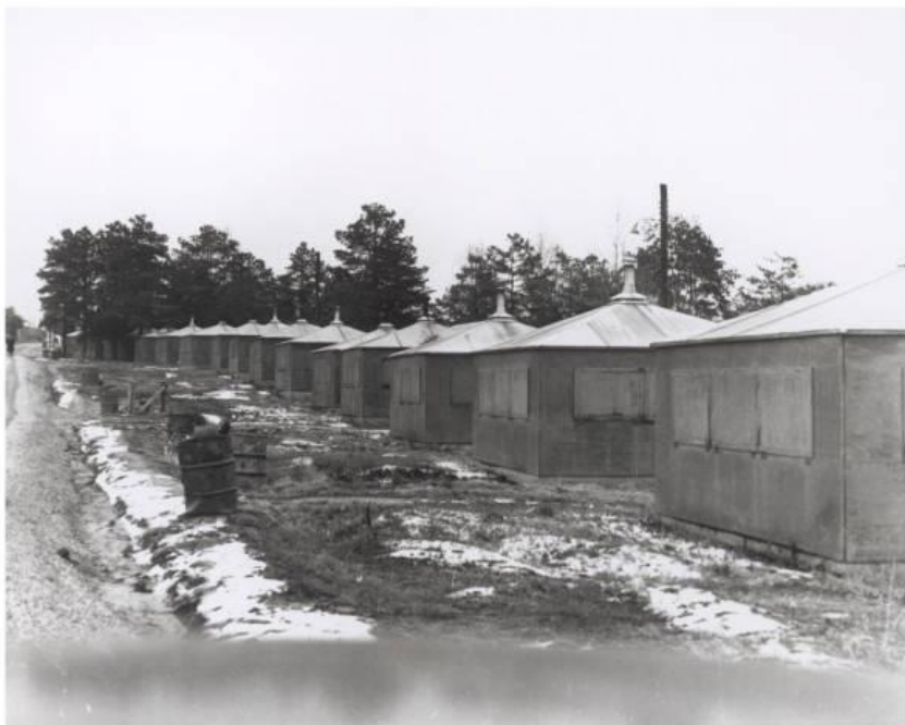
Figure 10: A row of hutments (Credit: DOE, ORPL)
