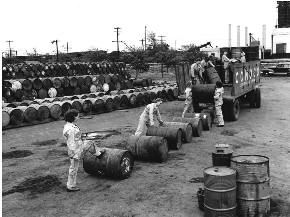
Figure 6: Ponca City Refinery, Conoco / Continental Oil Company, c.1942-44. (Courtesy of Phillips 66)
