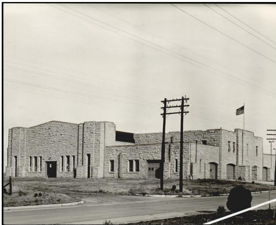
Figure 5: Tonkawa Armory in 1942, the location of the NYA Tonkawa radio training program. With Navy recruits joining the radio training, the NYA expanded to also include nearby buildings. [Photograph 2012.201.B1292.0011]; The Gateway to Oklahoma History , Oklahoma Historical Society.
