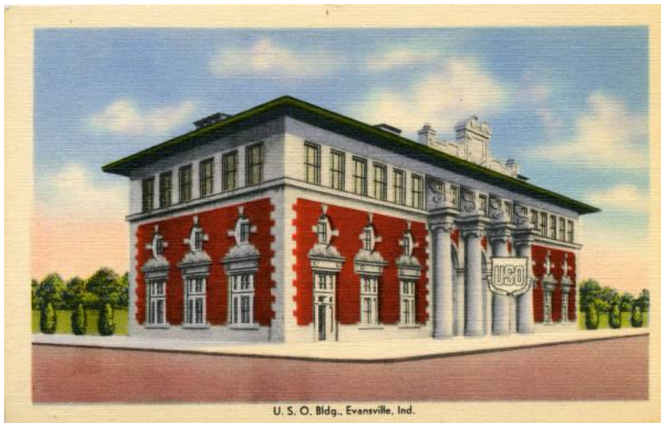
Figure 15: USO Club in Evansville, Indiana (1943), Eighth and Main Streets, formerly the Evansville and Terre Haute (E & TH) Railroad depot. (Credit: University of Southern Indiana, Rice Library Digital Collections)
