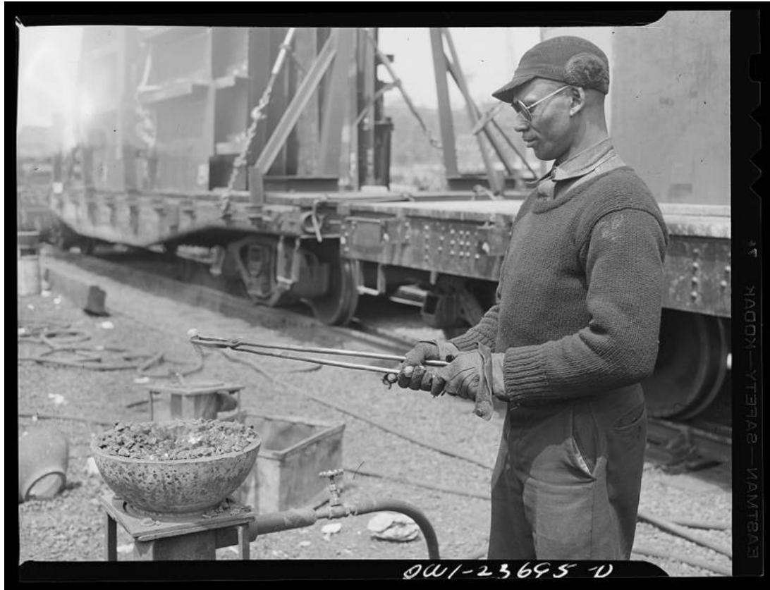
Figure 11: Bethlehem-Fairfield shipyards, Baltimore, Maryland. Heating Rivets. May 1943. (Credit: Arthur S. Siegel, Library of Congress)
