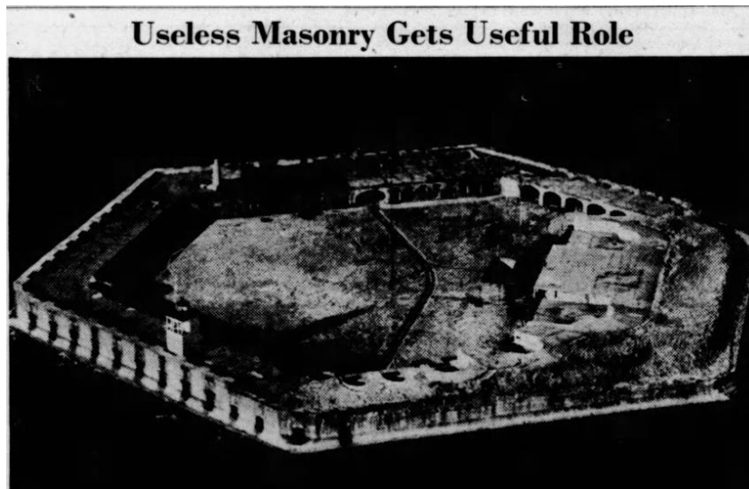
Figure 15: "Useless Masonry Gets Useful Role," is the title for a picture of Fort Carroll. The construction of the fort had been led by Robert E. Lee beginning in 1848. The picture was alongside text used for this lesson's quotation to consider. (The Baltimore Sun, Dec. 31, 1941)
