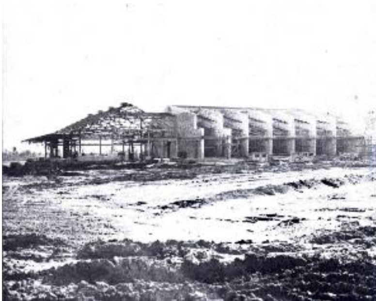
Figure 3: A photo of construction of the Shumaker Naval Ammunition Depot, in a 1950s publication by the depot: "NAD Yesterday and Today." (Courtesy of Public Library of Camden, Ouachita County)
