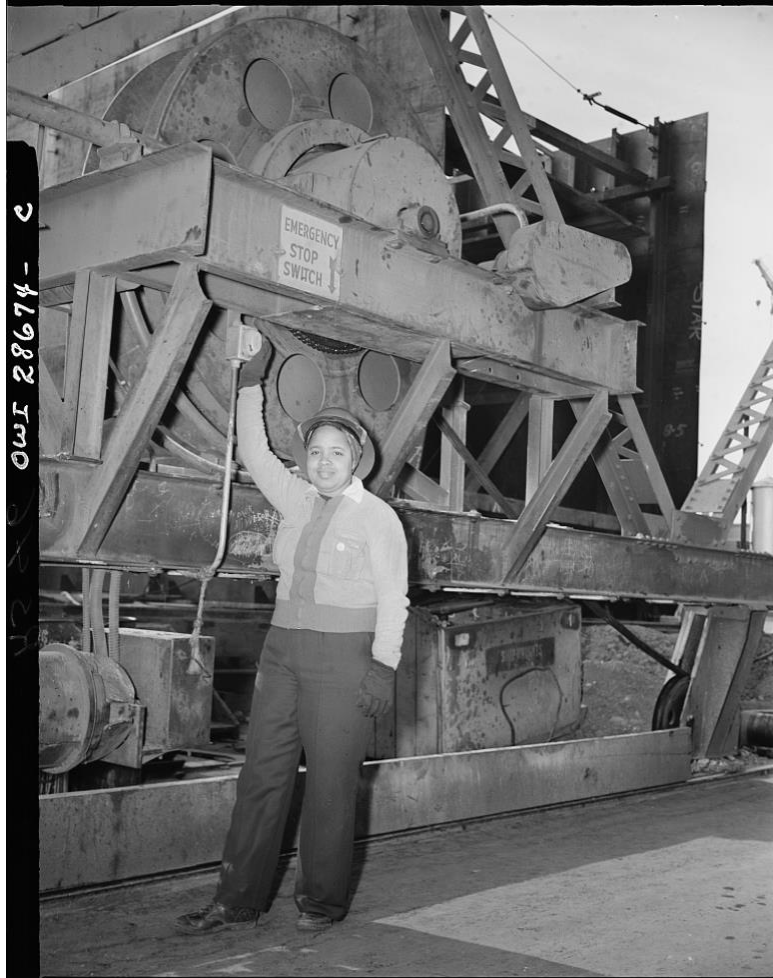
Figure 22: “Miss Odie Mae Embry mans the emergency switch for the protection of track workers as the huge crane swings 100 feet above...” to help construct SS George Washington Carver in Kaiser Shipyards. (Credit: Joseph, E. F., Library of Congress)
