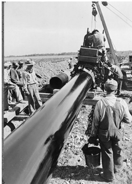
Installing Big-Inch Pipeline, 1944, Library of Congress, Prints & Photographs Division, FSA/OWI Collection
