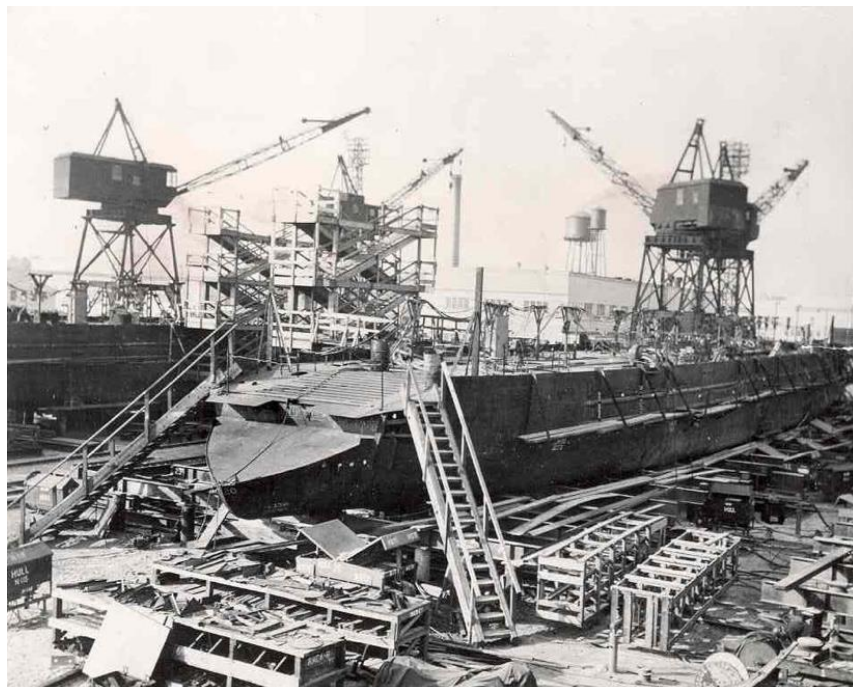
Figure 4: Landing Ship, Tank (LST) under construction at the Dravo Shipyard in Wilmington, DE during WWII (Credit: City of Wilmington)
