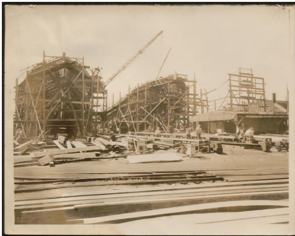
Figure 17: American Car & Foundry Co. yards, showing ships under construction in 1944. (Courtesy of the Hagley Museum and Library) 5
