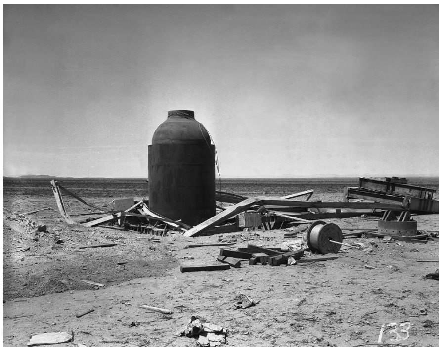
Figure 9: "Jumbo" and a collapsed tower after the Trinity Test. Jumbo was designed to hold the "Gadget" to save plutonium. It was deemed unnecessary and suspended from a tower during the Trinity test. It survived the explosion. (Credit: Atomic Heritage Foundation)
