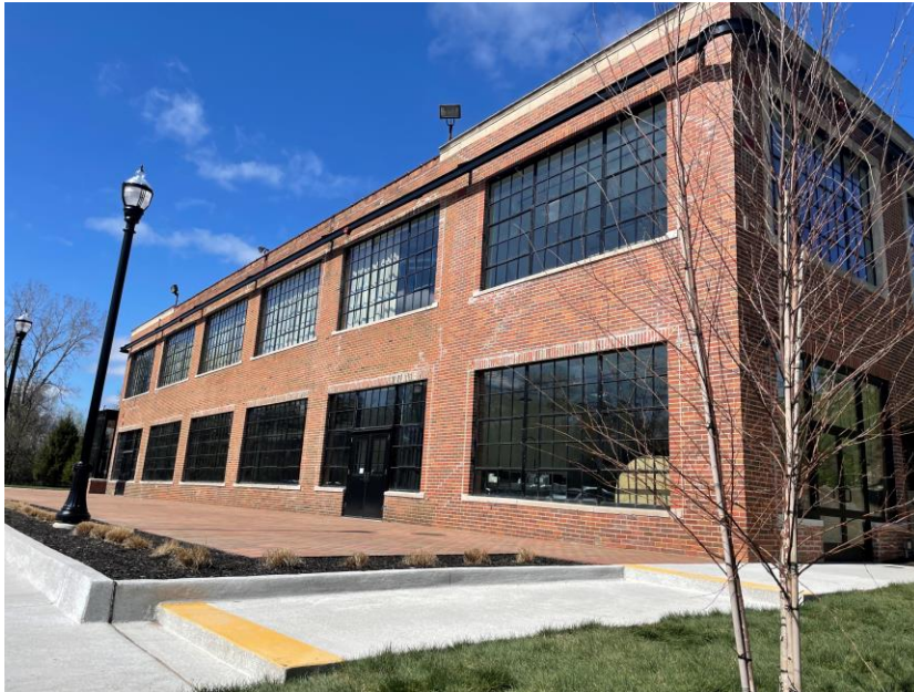
Figure 8: Today, the restored Phoenix Mill building is used as an event center. On the outside of the building you can see the steel railing that was used for blackout curtains during the war, as described in Reading 3. (Credit: Phoenix Mill Events)
