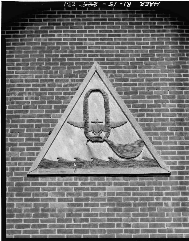
Figure 5: A close up of an exterior wall of enlisted barracks with a triangular wood Quonset Point Insignia. The buildings were designed by Albert Kahn, Inc., architects. (Historic American Engineering Record - Library of Congress)
