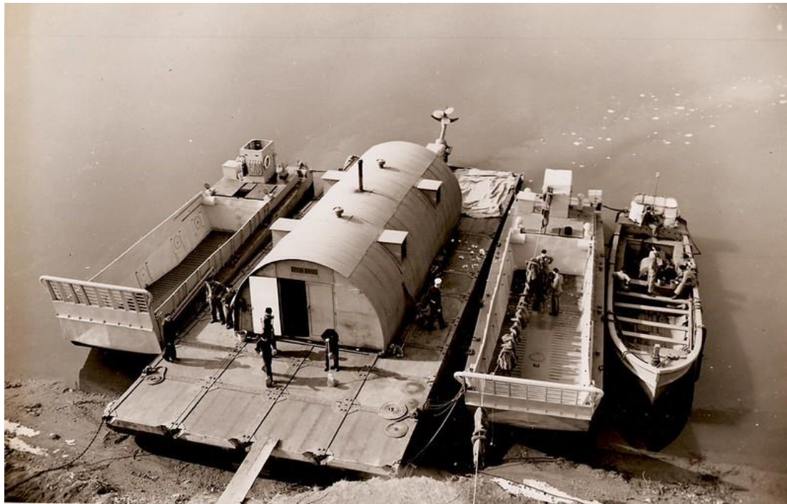
Figure 6: A Quonset Hut, designed in North Kingstown, Rhode Island, in use with Seabees training at the Seamanship school at Camp Endicott. These huts were built as temporary structures across the world during the war. (Courtesy of the United States Navy Seabee Museum Archive)
