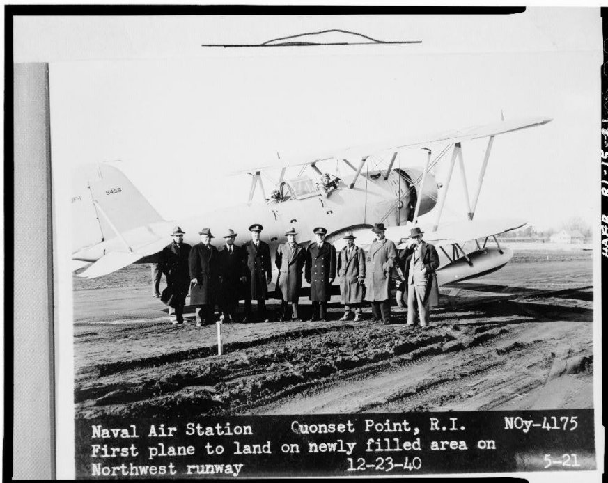
Figure 3: Naval Air Station – Quonset Point, R.I. - First plane to land on newly filled area on the Northwest runway, December 23, 1940. (Historic American Engineering Record - Library of Congress)
