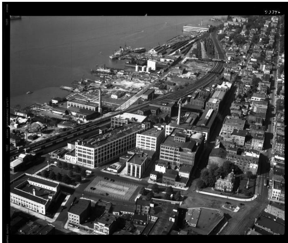
Figure 14: Aerial of buildings owned by the Otis Elevator Company in Yonkers. Railroad tracks, ships in port, and the Hudson River are also in view. The Company contributed to wartime manufacturing. (Source: New York State Archives, Aerial photographic prints and negatives of New York State sites, 1941-1957, B1598-99. Box 8, no. 65.)
