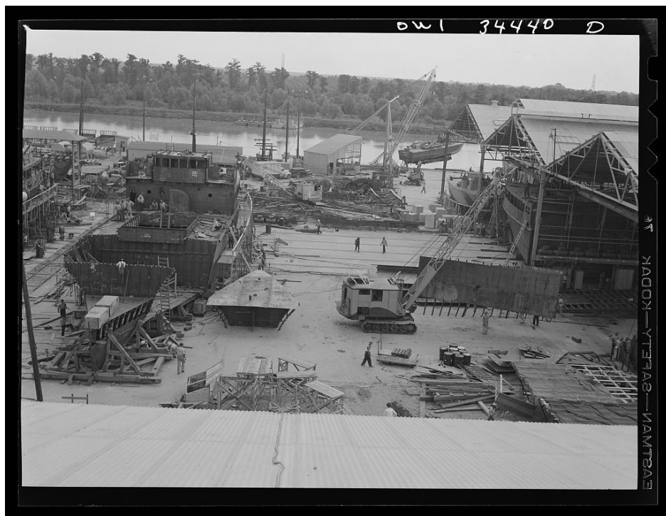
Figure 2: "Higgins shipyards, New Orleans, Louisiana. Cargo vessel under construction." June 1943. Photo by John Vachon, Office of War Information. Credit: Library of Congress.
