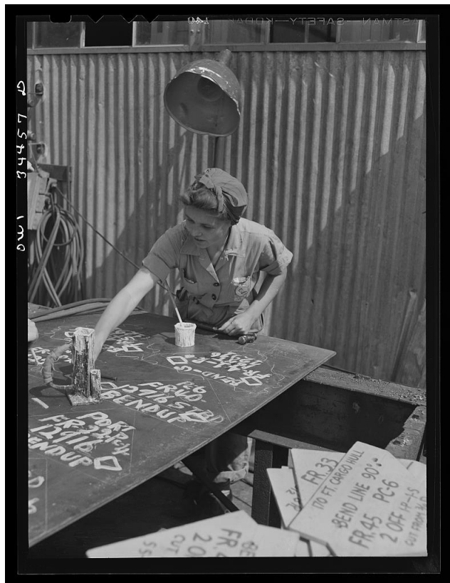
Figure 4: "Numbering steel plates ready for installation. Higgins shipyards, New Orleans, Louisiana." June 1943. Photo by John Vachon, Office of War Information. Credit: Library of Congress.
