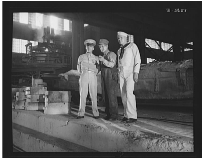
Figure 9: "A poster comes to life. 'Now, over there is...' For six days, Woolslayer acted as guide for his Army and Navy companions and even then failed to cover the entire mill. Note, in left background, an electric furnace in operation. Allegheny-Steel, Pittsburgh, Pennsylvania," August 1942 (Credit: Palmer, Alfred T., photographer; United States Office of War Information; Library of Congress)
