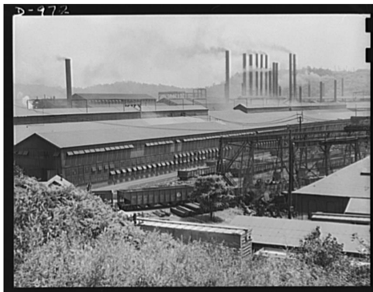
Figure 2: "Steel alloy manufacture. Allegheny Ludlum Steel Corporation, Brackenridge, Pennsylvania. General view of part of the plant where scrap iron and steel are converted into many grades of steel alloys. In the foreground are carloads of finished products, while in the middle foreground can be seen piles and cars of scrap coming in to feed the huge furnaces. In the background is the power house which supplies electricity and steam to turn the wheels of this important defense industry, set in the Pennsylvania hills about thirty miles north of Pittsburgh, one of America's most important steel producing centers" (Credit: Alfred Palmer; Library of Congress)
