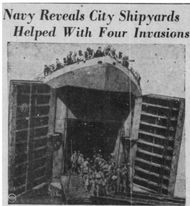
Figure 2: "Navy Reveals City Shipyards Helped With Four Invasions." The photo shows a tank landing craft like those made in Wilmington. The ship shows how the bow opens to receive and discharge cargo. In this photo, troops are using it to go to the fighting front. (Journal-Every Evening, Oct. 2, 1943)
