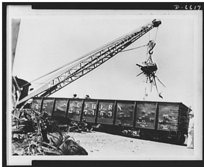
Figure 21: "Salvage. Scrap metal. The magnet loader of a large Southern junkyard operates continuously to keep our steel mills supplied with the scrap metal needed to make the tools of war. Location: in a large New Orleans yard." June 1942. Photo by Hollem Howard, Office of War Information. (Credit: Library of Congress)
