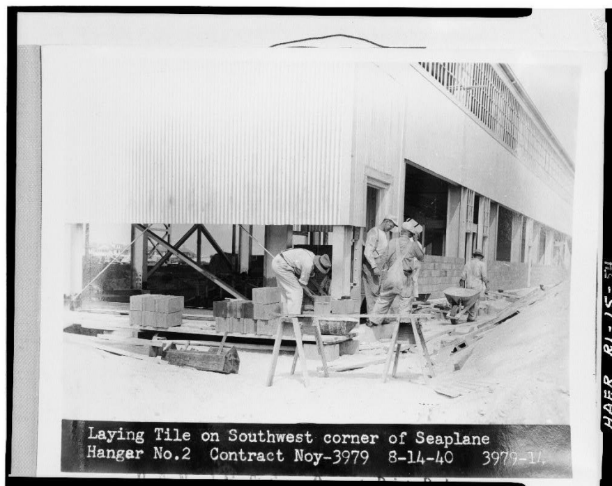
Figure 2: "Laying Tile on Southwest corner of Seaplane Hangar No.2, 8-14-40 (Historic American Engineering Record - Library of Congress)
