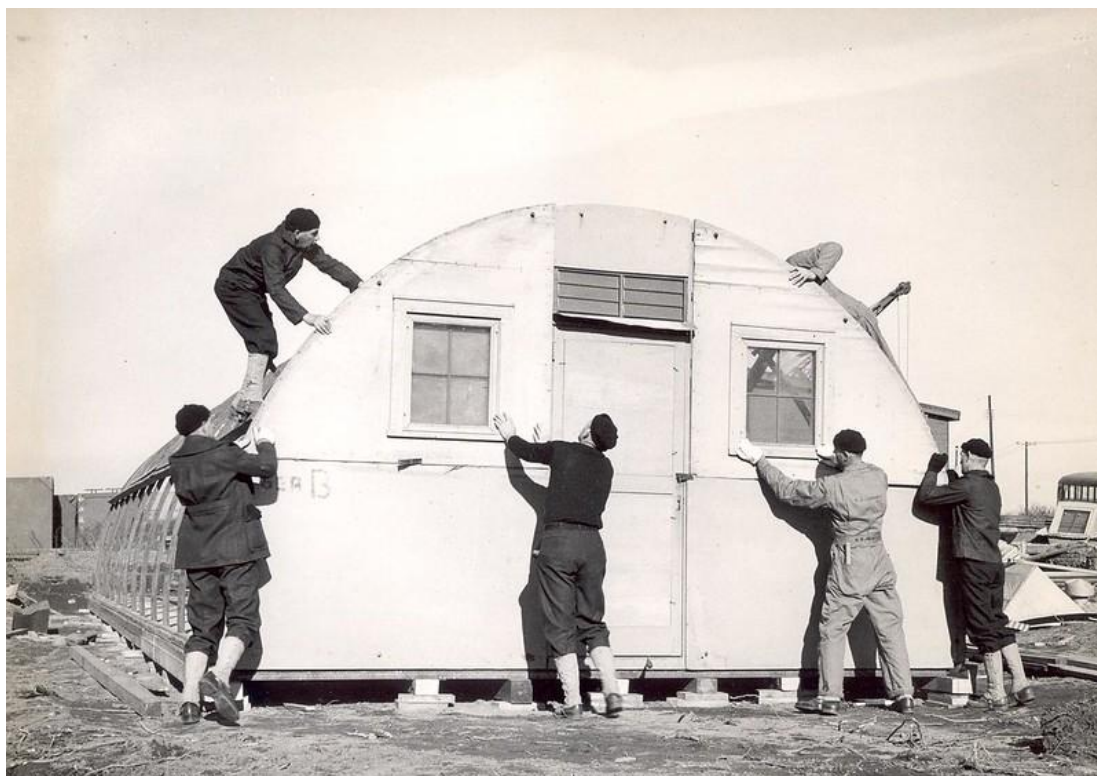
Figure 7: Seabees constructing a Quonset Hut as part of their carpentry training at Camp Endicott in Davisville in 1942. (Courtesy of the United States Navy Seabee Museum Archive)
