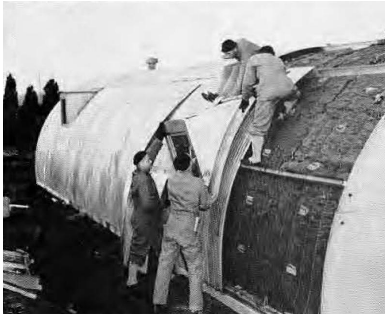
Figure 21: Seabees constructing a Quonset Hut. From a Camp Endicott yearbook by the U.S. Navy Department, Office of Public Relations.
