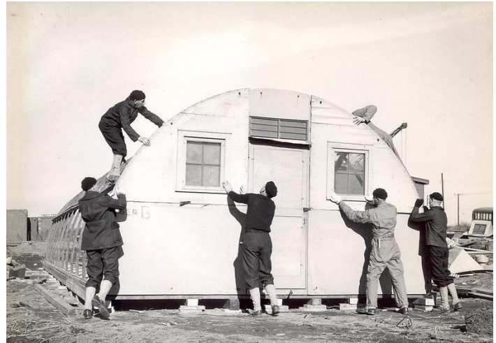
Seabees constructing a Quonset Hut as part of their carpentry training at Camp Endicott in Davisville in 1942. Courtesy of the United States Navy Seabee Museum Archive
