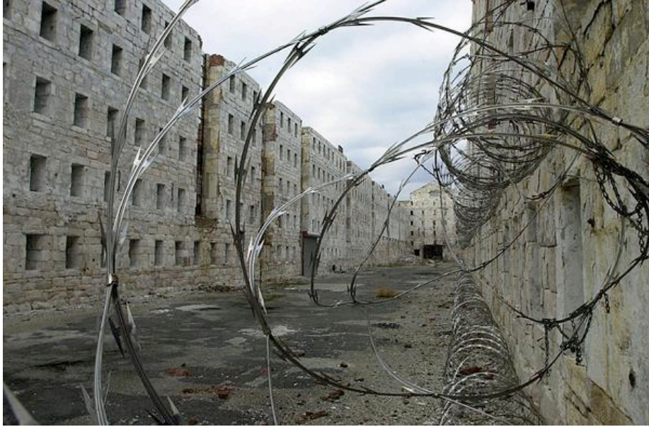
Fig. 1. Original Cellblock's current condition.
