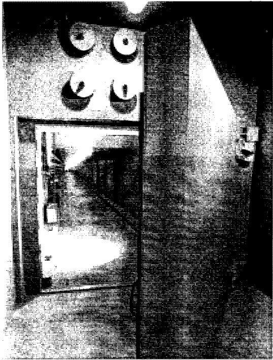
Blast door entrance to the Cold War bunker located under The Greenbrier.
